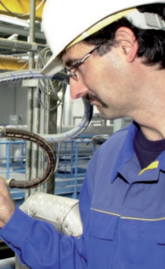
Monitoring of industrial systems; here the visual inspection of a safety valve.
