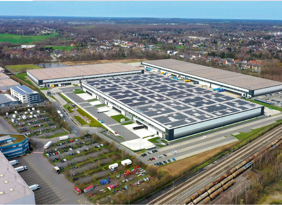
SEGRO Logistics Park Oberhausen
